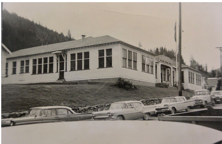
View of office in 1950s, Bridge River Valley Community Association
