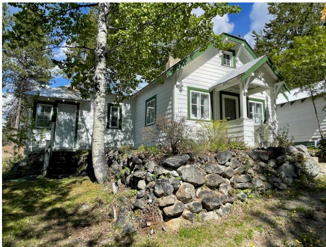
Front view of teacherage in 2021, Bridge River Valley Community Association
