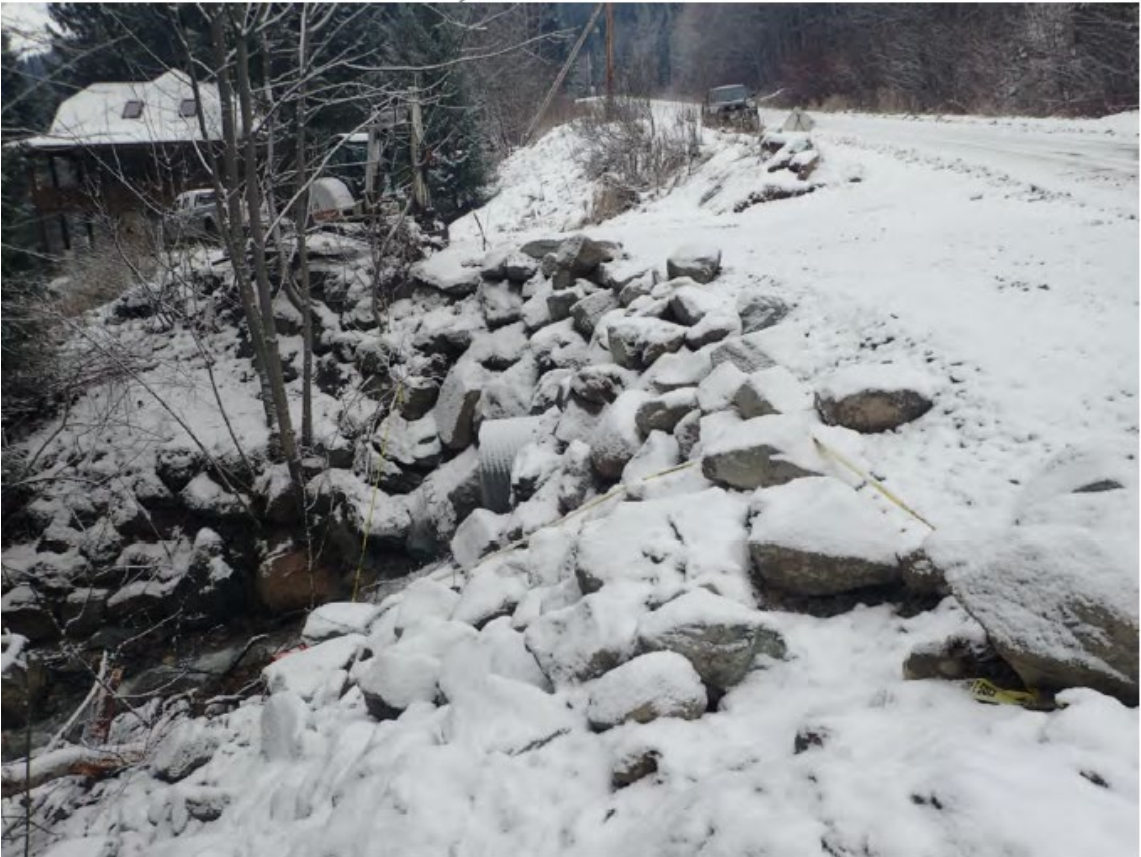
Reid Road Culvert (December 12, 2021) Cordilleran (December 13, 2021)
