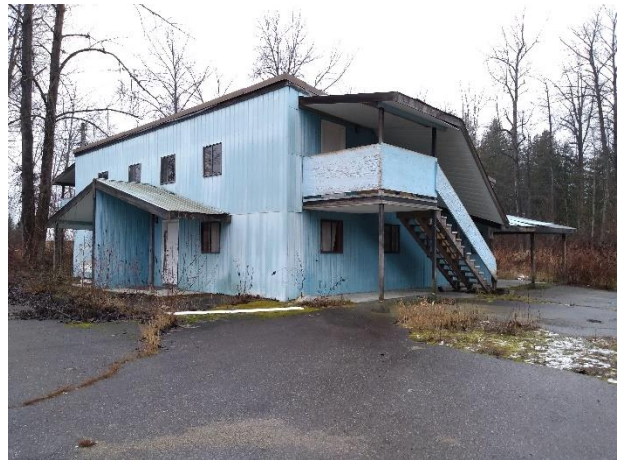
Photo 16: Lot B vacant 2 story dwelling and asphalt paving. December 13, 2019.
