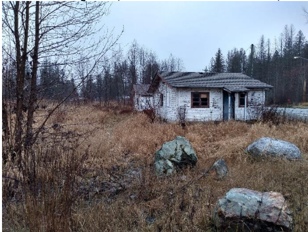
Photo 17: Lot B small vacant residential buildings. December 13, 2019.
