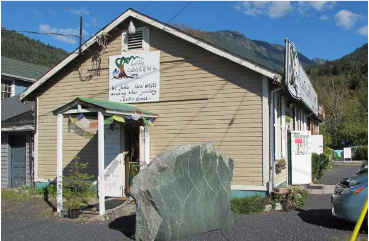
Dining Room & Bunkhouse, 2018
