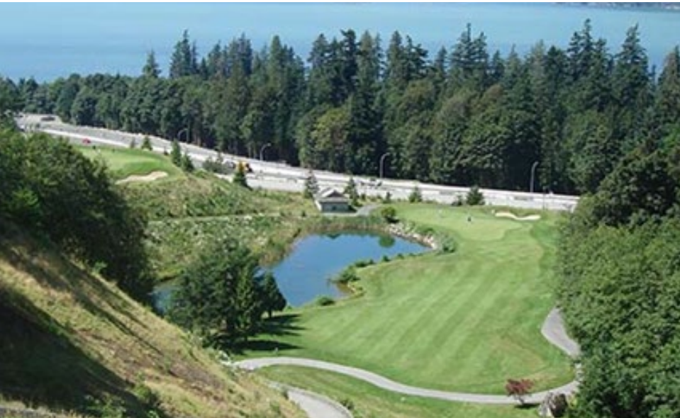
A new lake adjacent to the golf course's 1 st hole serves as a part of the community's stormwater management system.
