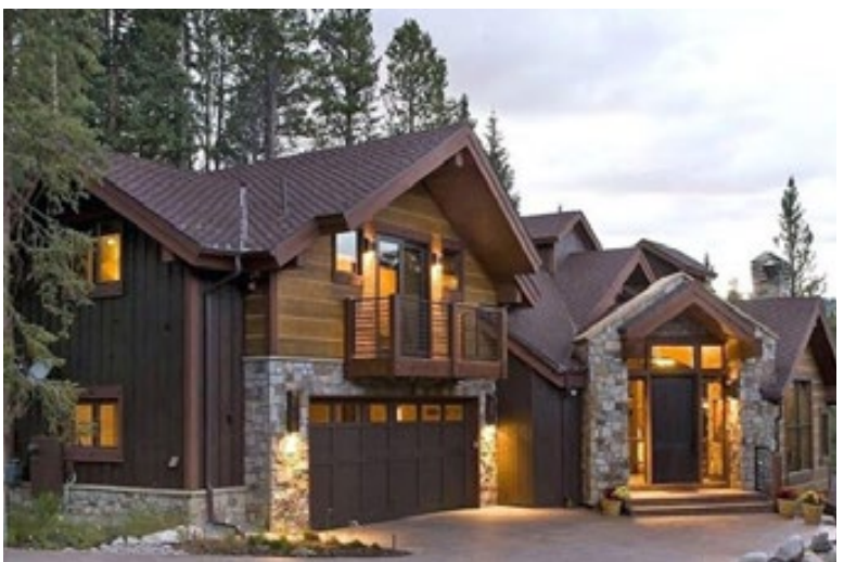
Stone and siding, local materials
