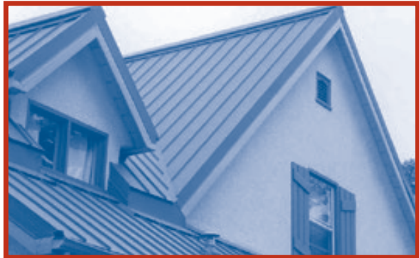
Metal, clay tile, asphalt shingles, or non-combustible material (0 pts) - the most fire resistant and remain effective under severe fire exposure.
