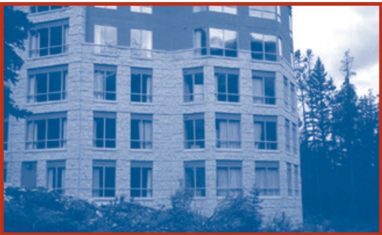
Non-combustible siding (0 pts) Materials such as stucco, metal siding, brick cement shingles, concrete block, poured concrete, and rock offer superior fire resistance.
