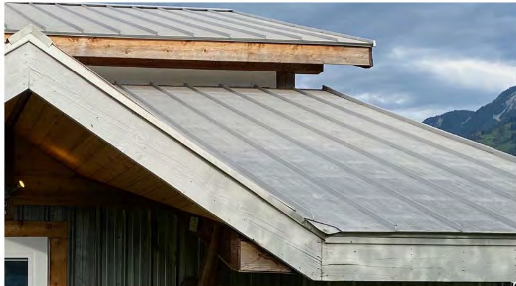
3 standing seam metal roof, wood fascias
