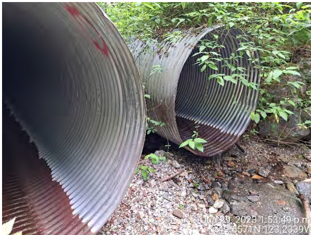
Photo 13: Culverts (~2 m diameter) that convey Unnamed Stream 1 under highway 99 onto the subject site.
