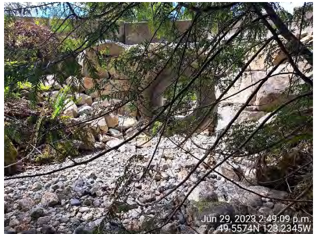
Photo 14: Looking west (downstream) at the large culvert that conveys Unnamed Stream 1 under the gravel access road for the aggregate quarry on the subject site.
