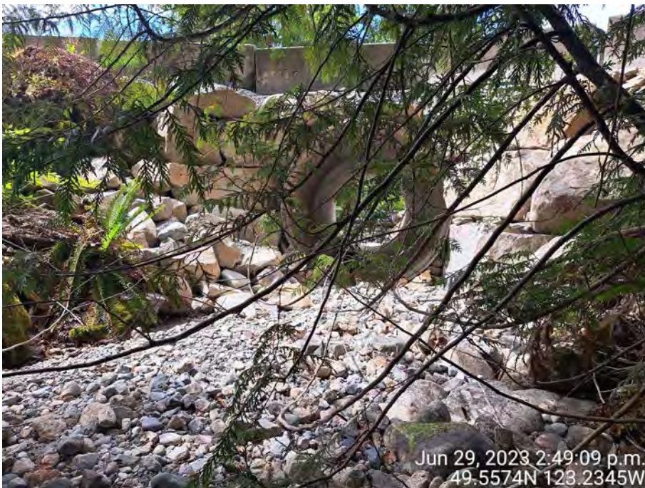
Photo 4: Looking downstream at the large culvert (~2.8 m diameter) that conveys Unnamed Stream 1 under the gravel access road for the aggregate quarry on the Property.
