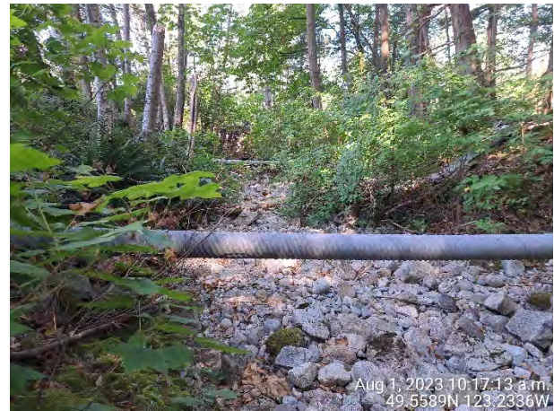
Photo 20: Looking west (downstream) at the two water pipes crossing Unnamed Stream 2.
