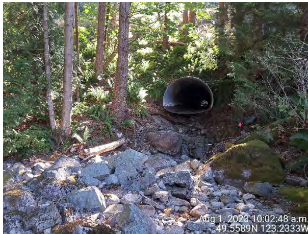
Photo 19: Looking east (upstream) at the large culvert that conveys Unnamed Stream 2 under Highway 99.
