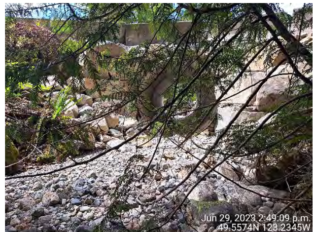
Photo 6: Looking west, downstream, at Polygon 3, the watercourse as it flows through the central culvert on the subject site. June 29, 2023.
