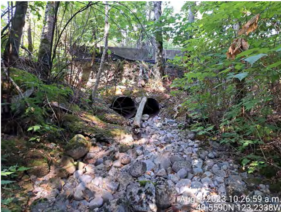
Photo 12: Looking west (downstream) at the culvert that convey Unnamed Stream 2 under the Property access road, the railway tracks, and the Provincial Park access road.
