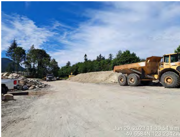
Photo 23: Looking south at aggregate quarry activities on the subject site. June 29, 2023.
