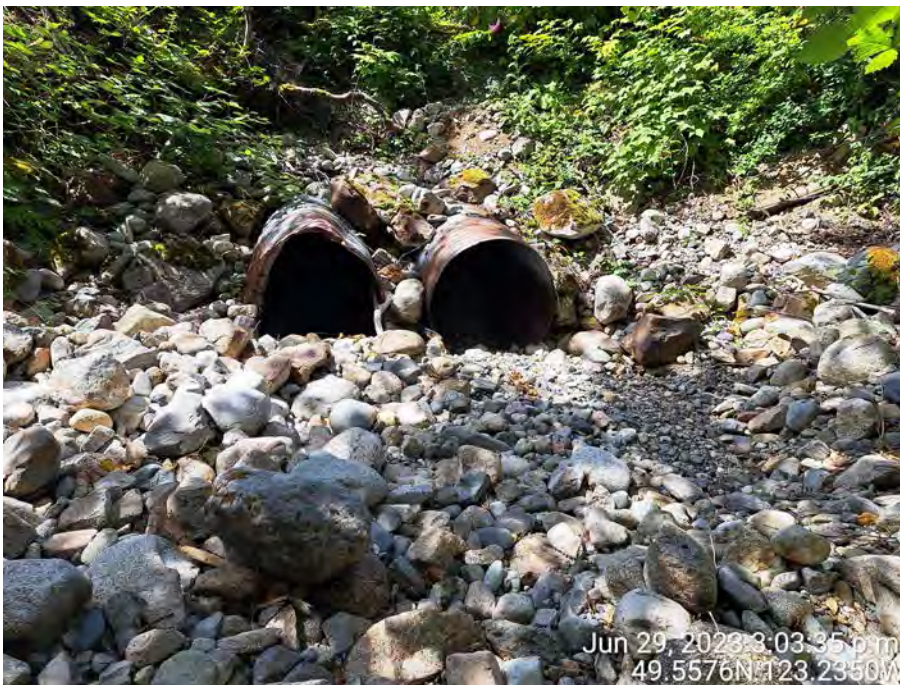
Photo 6: Looking downstream at two culverts (~0.8 m diameter) that convey Unnamed Stream 1 under a gravel access road on the Property and the railway tracks, located off Property.
