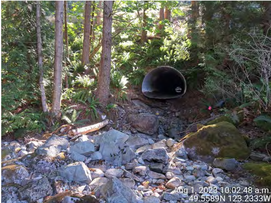
Photo 9: Looking east (upstream) at the large culvert that conveys Unnamed Stream 2 under Highway 99.
