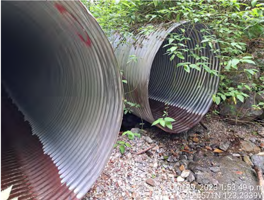
Photo 1: Culverts (~2 m diameter) that convey Unnamed Stream 1 under highway 99 onto the Property.
