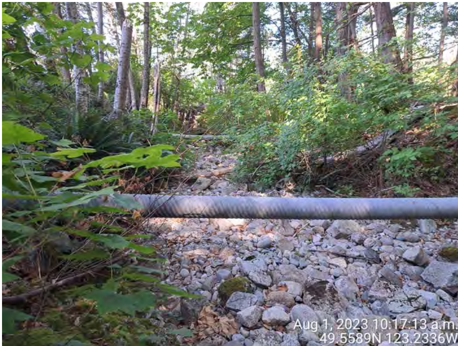
Photo 11: Looking west (downstream) at the two water pipes crossing Unnamed Stream 2.
