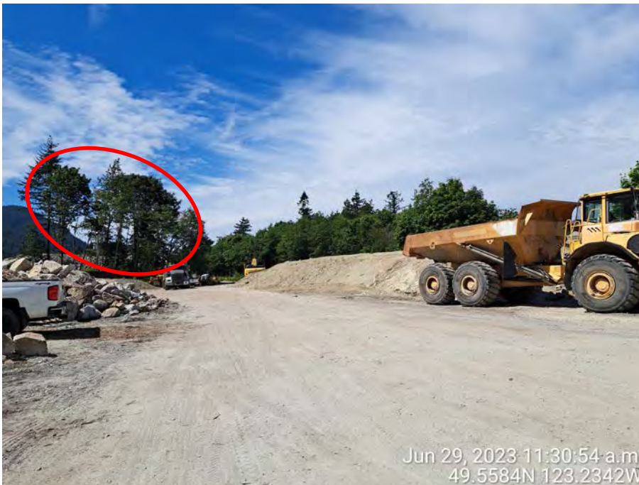
Photo 8: Looking south at the aggregate quarry activities on the Property. The trees circled in red are the only riparian trees remaining within the Unnamed Stream 1 SPEA at the stream's downstream extent.
