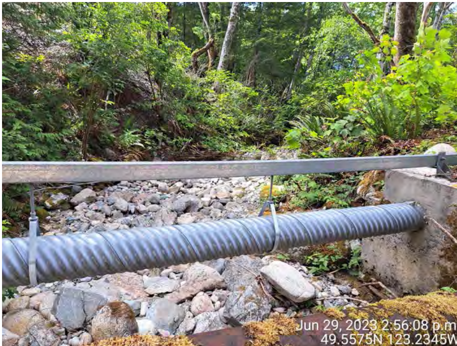
Photo 5: Looking downstream at water pipes crossing Unnamed Stream 1 on the Property that convey drinking water to the neighbouring provincial park to the west of the Property.
