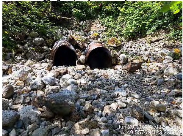
Photo 16: Looking west (downstream) at two culverts that convey Unnamed Stream 1 under a gravel access road on the subject site and the railway tracks, located offsite.
