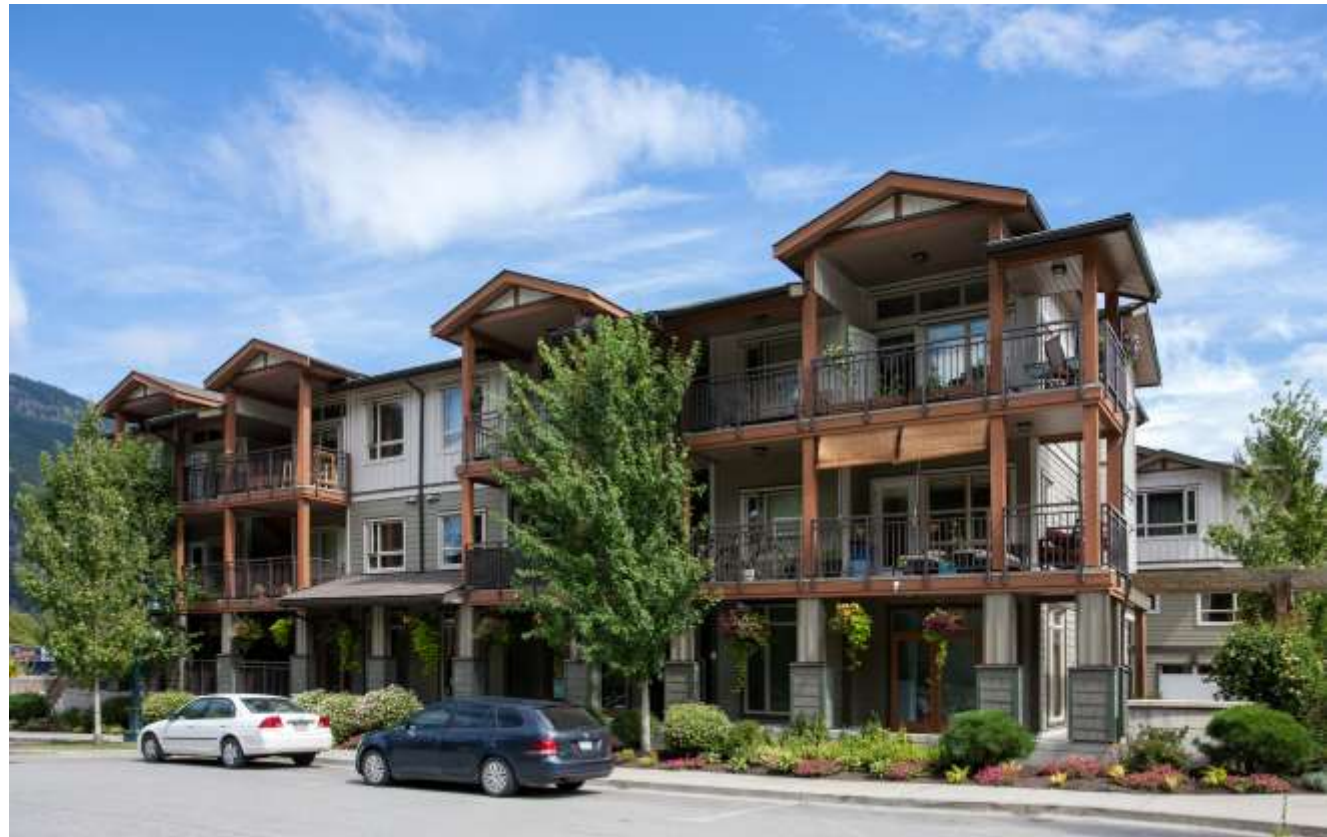
Expedition Station is a mixed use development with 17 condos above four small commercial units. The Westcoast-inspired homes offer private patio spaces and secure garages, and the top floor units have vaulted ceilings.
