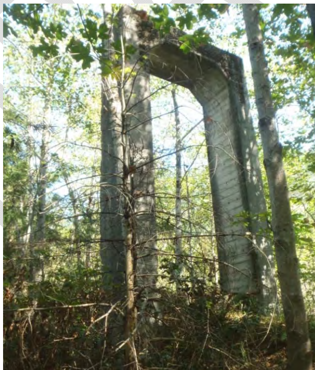
Photo 10. Concrete foundation of former Britannia Mine elevated roadway structure.
