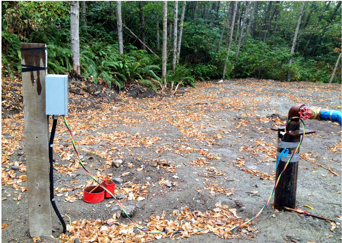
Photo 2. TW2 well head during pumping test, August 2, 2013.
