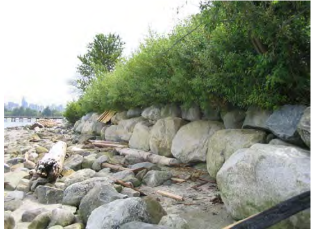
Photo 10: Example of coastal shoreline protection for larger waves using boulders and bioengineering.
