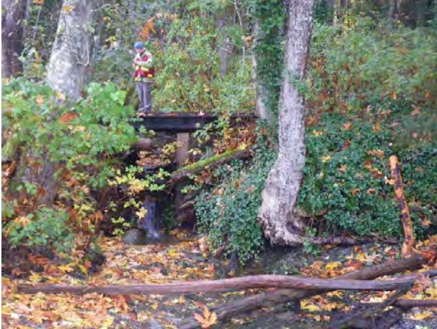
Photo 9: Unnamed Creek, looking upstream at ocean outlet (culvert under bridge).
