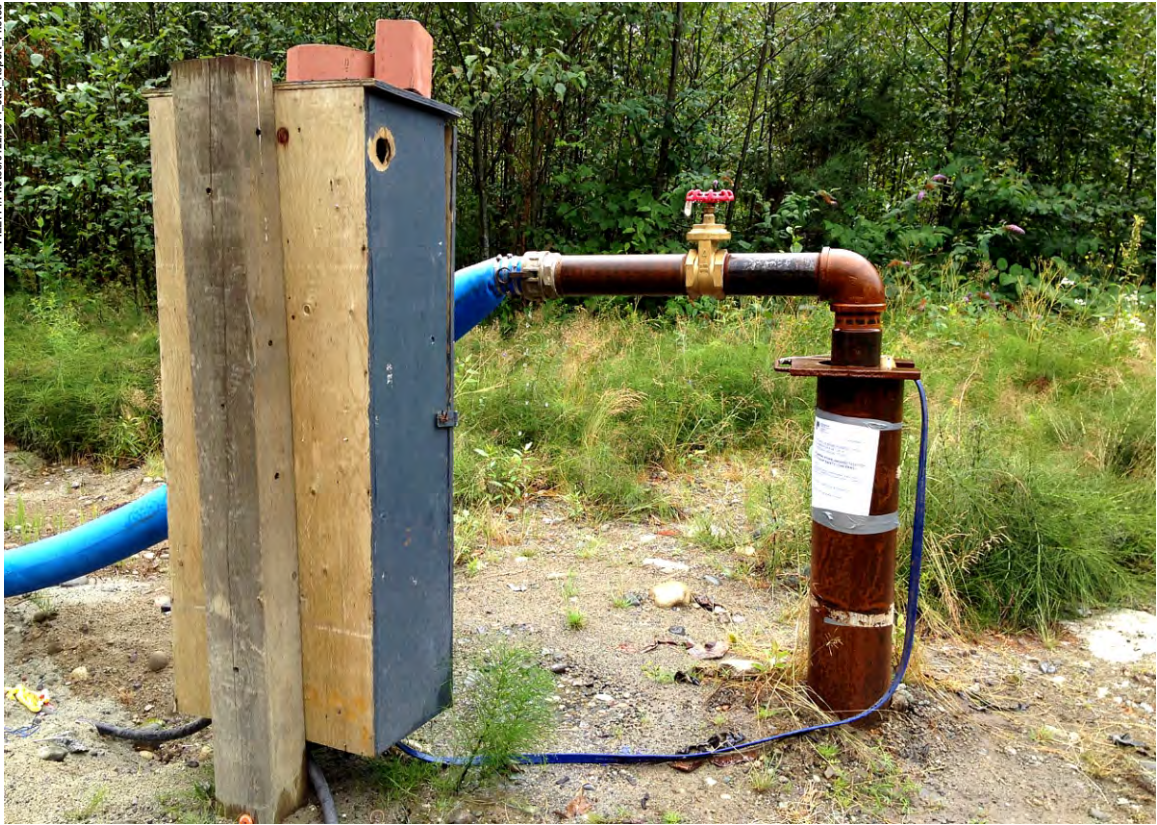
Photo 1. TW1 well head during pumping test, August 2, 2013.
