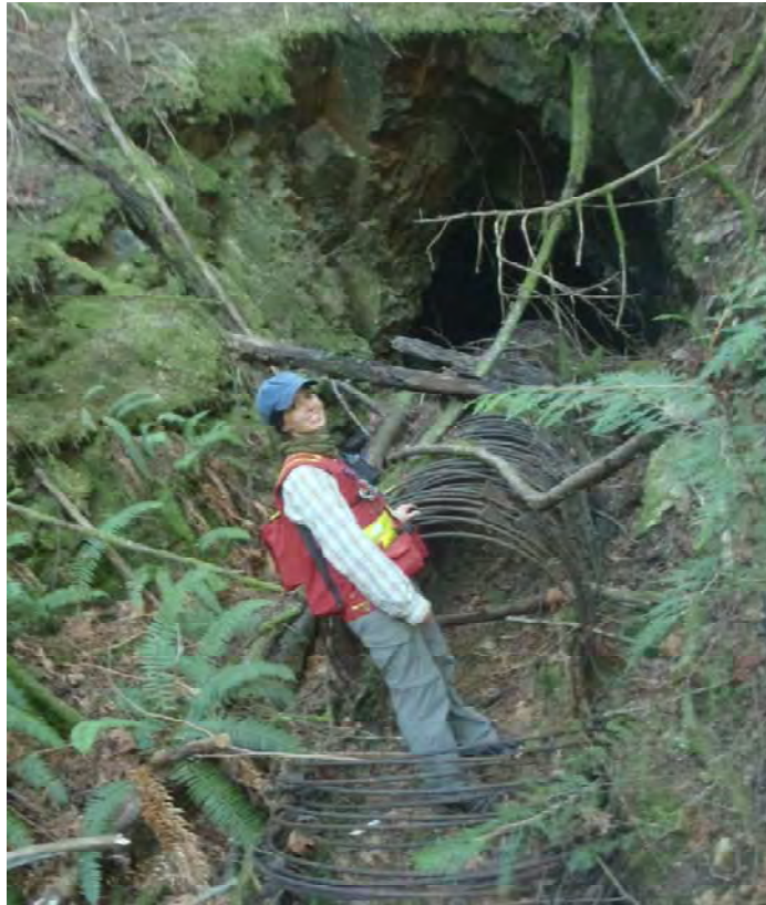
Photo 4. Waterline tunnel blasted through the rock near Thistle Creek in DL 3717.
