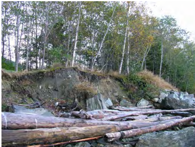
Photo 31: Eroded soil above the intertidal zone, shorezone unit A, November 4, 2011.
