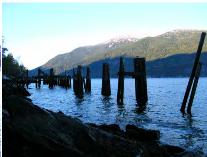
Photo 34: View of the old wharf pilings facing south, shorezone unit A, November 4, 2011.
