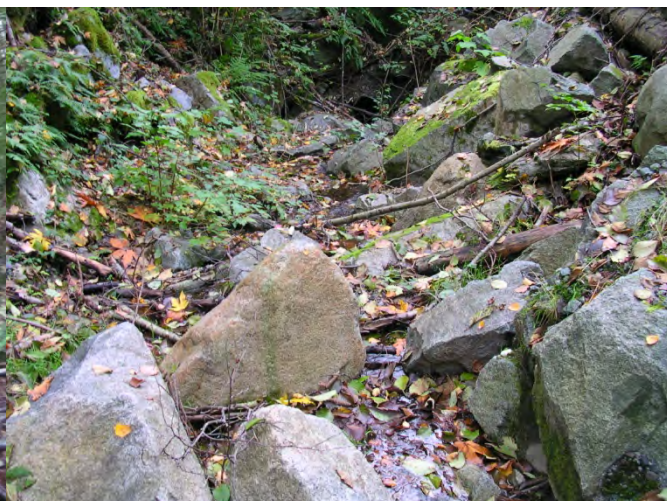
Photo 26: View of drainage 5 just upstream of the highway crossing culvert. Photo taken facing downstream.
