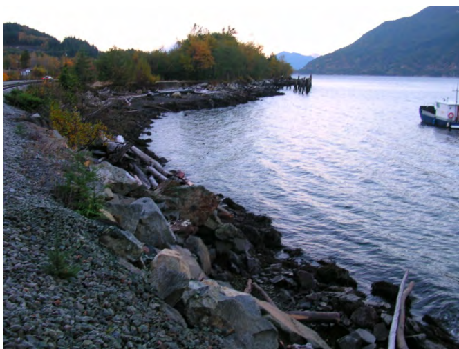
Photo 29: View of shorezone unit A from the northern property boundary facing south. Photo taken at 08:31, November 4, 2011.
