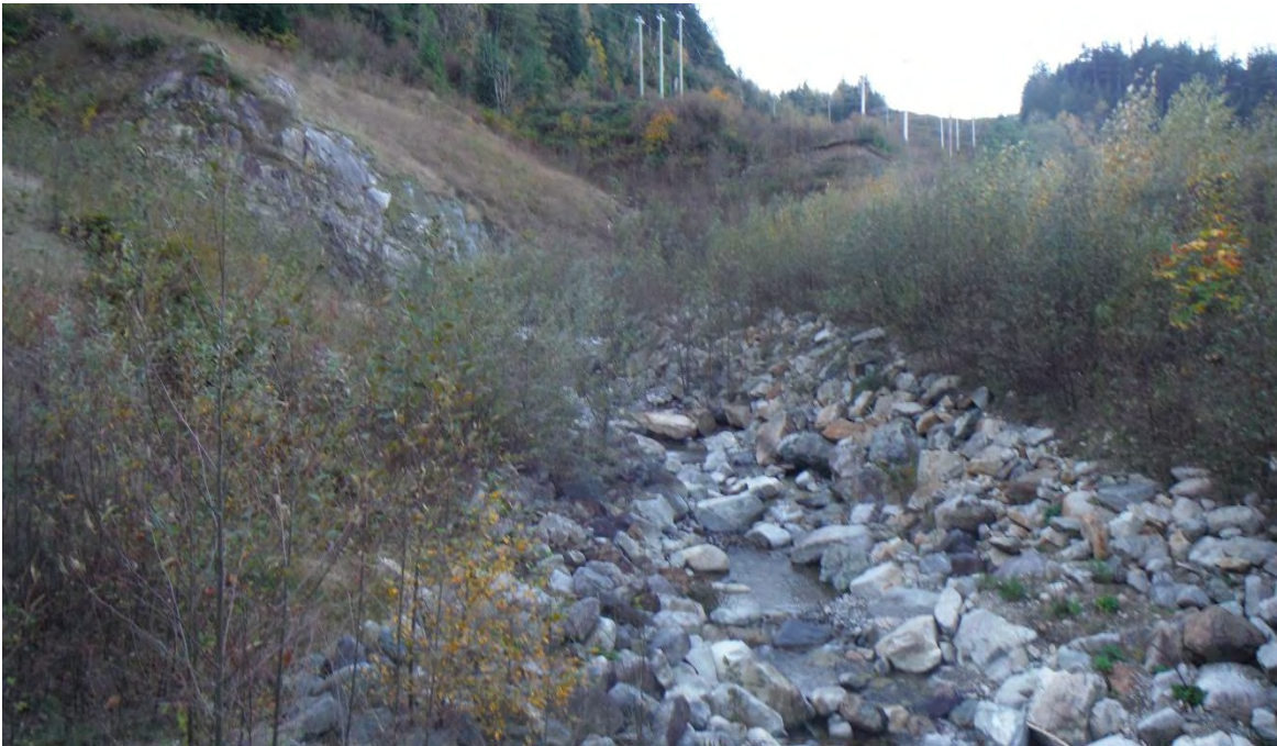
Photo 1: Debris Basin Looking Upstream from Spillway October 16, 2015
